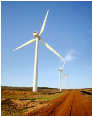
Darling wind farm
